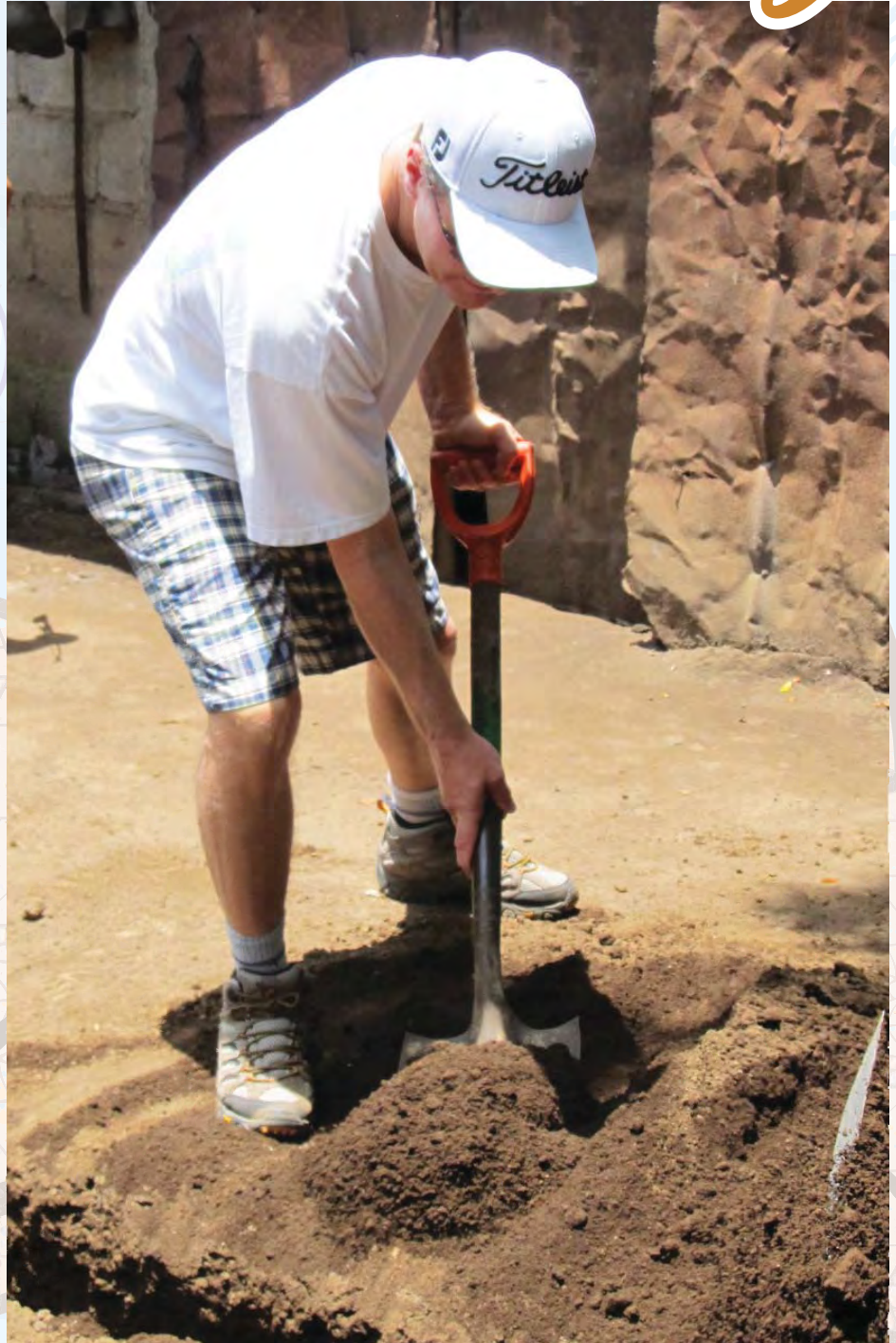
Darrell Borne digging a trench for an Amigos for Christ water project.
